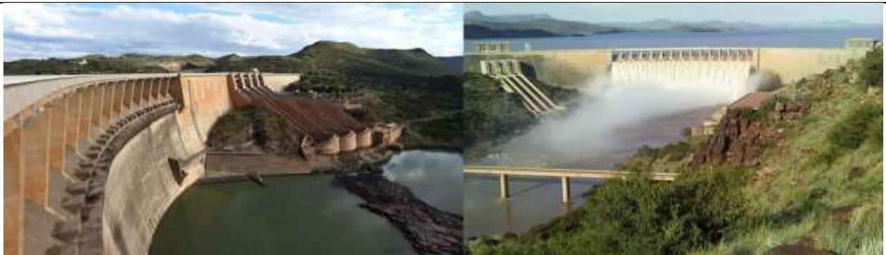
The Gariep Dam – Norvalspoor, Eastern Cape/Free State: The Gariep Dam forms part of the Orange River Development Scheme and is the largest hydro-electric dam in the country. Electricity from the dam is fed into the Eskom network at the Hydra Distribution Station near De Aar, which is one of the distribution stations fed by the transmission lines linking the Western Cape with the power stations in Mpumalanga.
